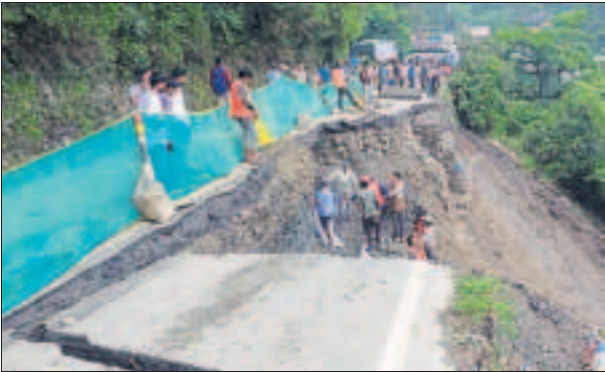
Repair work underway on the stretch of the Mussoorie-Dehradun road that subsided following heavy rain near Pani Wala Bend. HT
